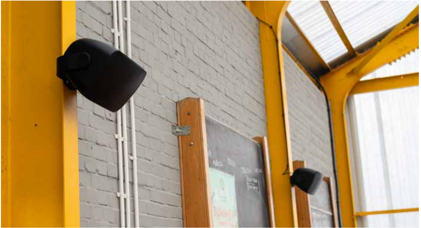
Four pairs of full-range Sonance Mariner 86 all-weather speakers handle the audio at The Hothouse events hub
